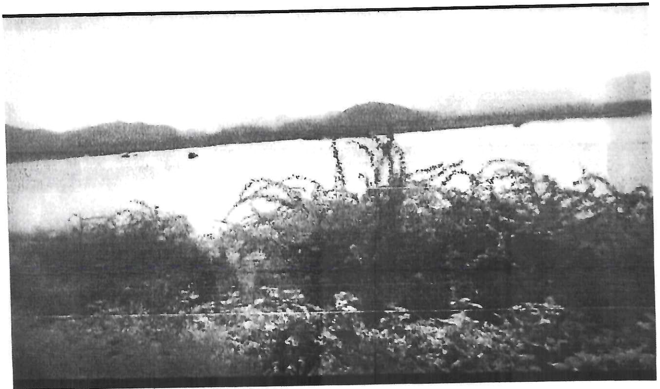
Raipur Patan dam
