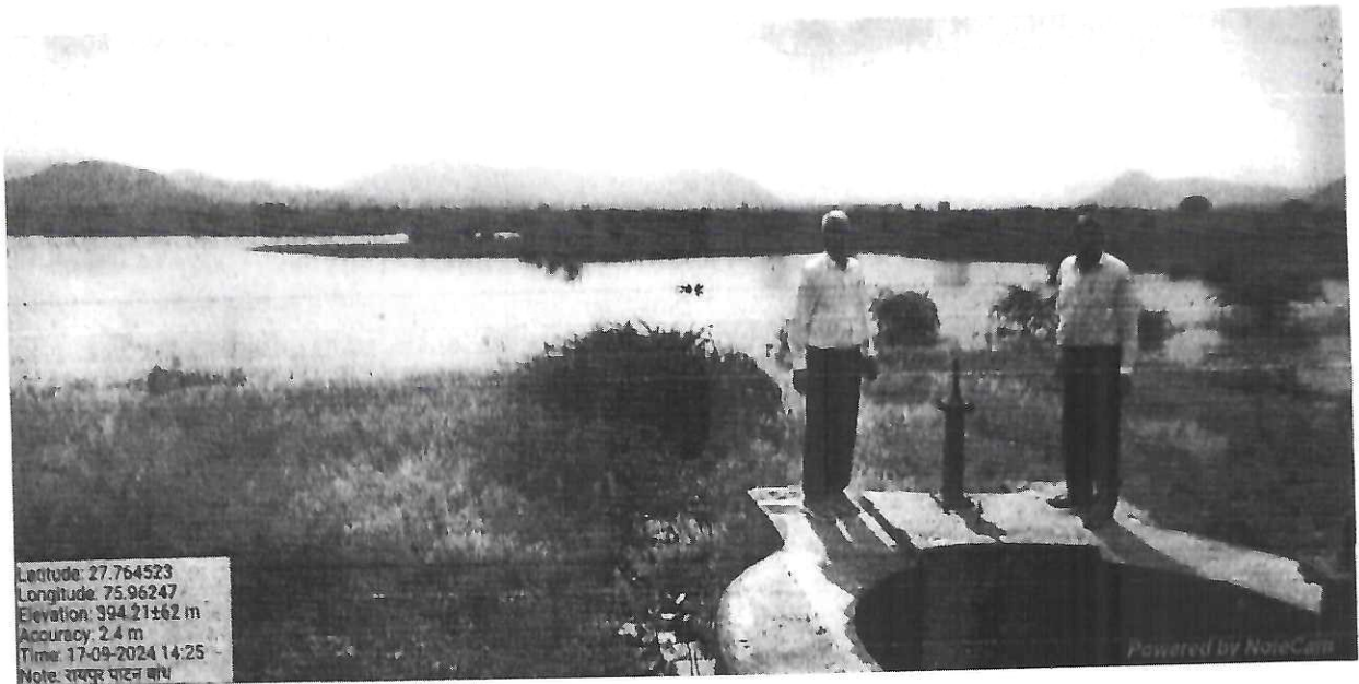
Raipur Patan dam
